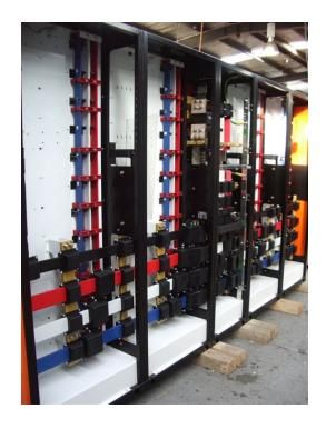
Rear of a switchboard showing busbars insulated by rigid sleeving and busbar joint covers
