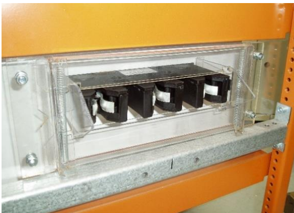
Busplug/tray partly inserted
